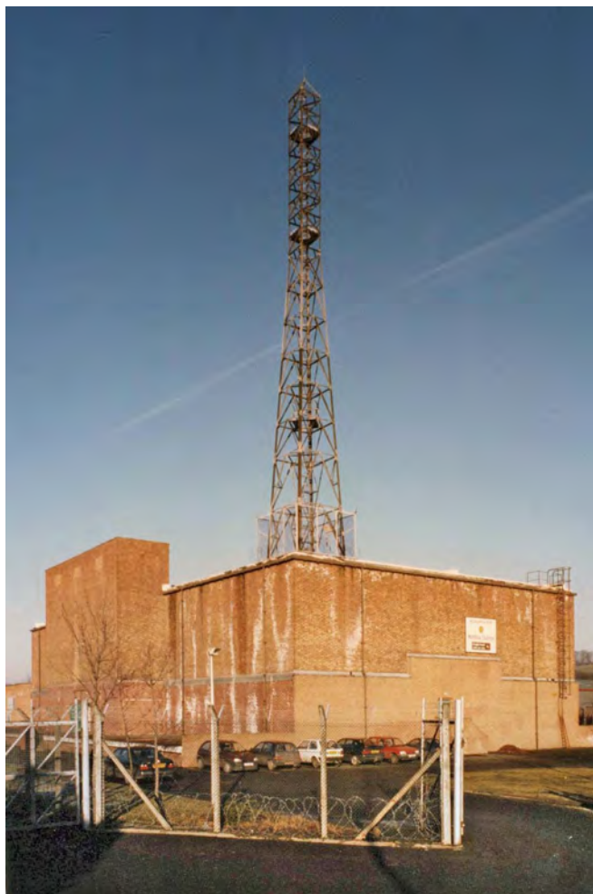
SRHQ 1.1 located in the cold store at Hexham in 1997. The building has now been demolished. Photo Richard Lamont The Home Office formally asked the PSA to proceed with the conversion in May 1983. Incidentally, the Home Office started to refer to the site as Zone Headquarters
